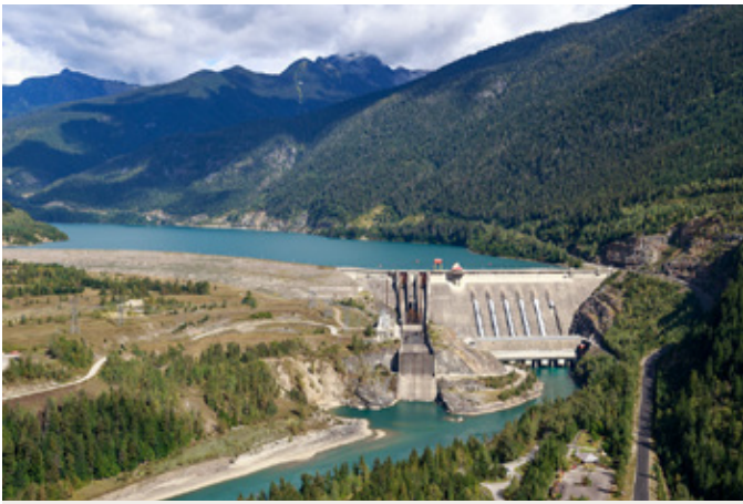
Revelstoke Generating Station
