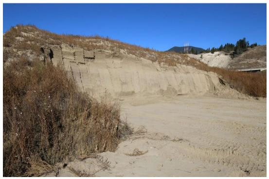
Figure 5. Substrate pile in Athalmer after resloping work had been completed by heavy machinery.
