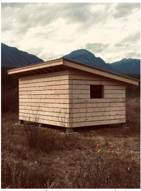
Figure 12. Artificial nesting structure for Barn Swallows built in Golden in 2023. 12'  $\times$  18' with slanted roof and low amount of openness.
